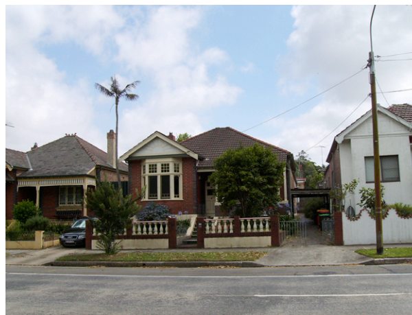
Figure 21.25 to 21.32. Frazer Street. This very good group has retained their original form, roofs (including slate roofs and slender chimneys) and attention to fine details such as timberwork, duochrome brickwork and tiling to stairs. Two have a form matching that found in Miller Street with a half-hipped hood to the front window, suggesting that the same builder was responsible.
