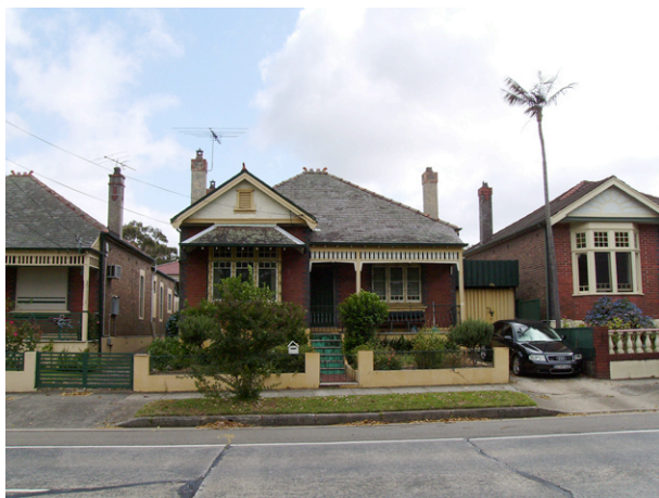
Figure 21.25 to 21.32. Frazer Street. This very good group has retained their original form, roofs (including slate roofs and slender chimneys) and attention to fine details such as timberwork, duochrome brickwork and tiling to stairs. Two have a form matching that found in Miller Street with a half-hipped hood to the front window, suggesting that the same builder was responsible.
