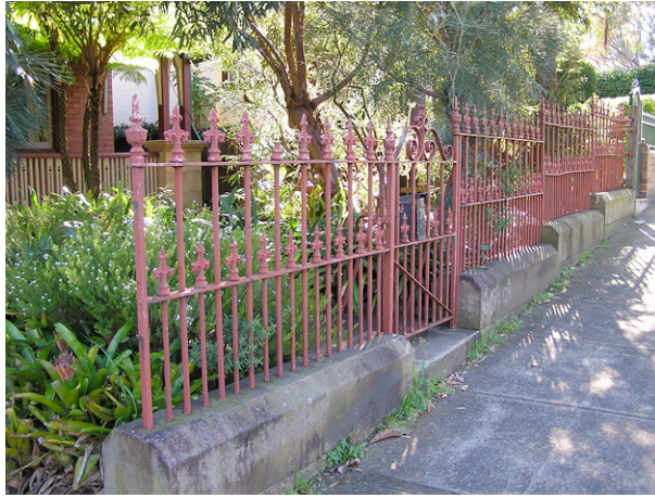
Figure 21.36. Detail of iron palisade fence set in chamfered base and stepping down to follow the slope of the hill
