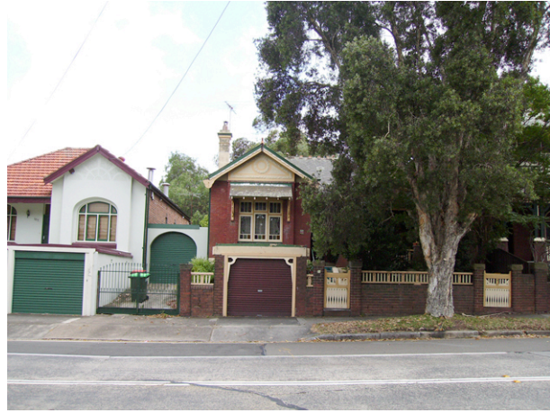
Figure 21.31 Frazer Street. This example follows the form common in this part of Marrickville, with the gable being an extension of the main roof, and the ridge forming an 'L' shape (see also HCA 29 – South Dulwich Hill.)
