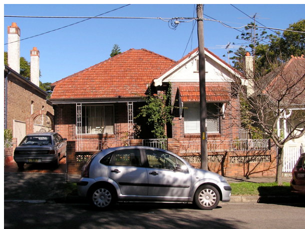
Figure 21.42. Replacement of timber joinery windows and veranda detailing with aluminium was a common form of layering in the 1970s and 1980s.
